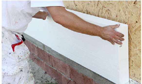
Figure 52: XPS installation on wall
