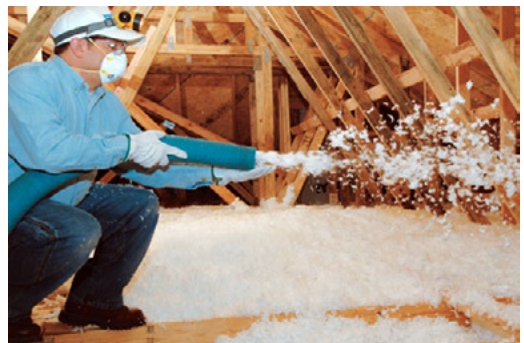
Figure 50: Insulation being blown-in
