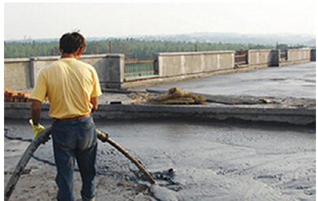
Figure 40: Foam concrete being applied as roof insulation
