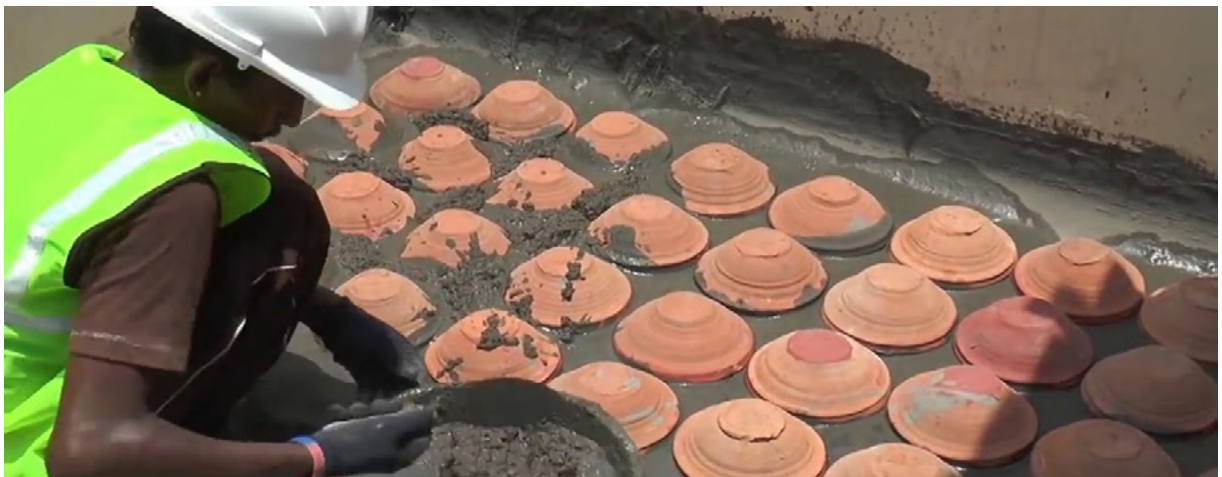
Figure 42: Inverted earthen pots insulation
