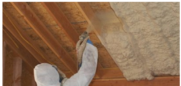
Figure 51: Foam insulation being blown-in
